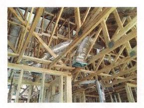
The air conditioning sub contractor comes in to install the supply lines, the supply boots where the grills will go, drain lines, service copper lines, and thermostat wires to desired locations.
