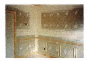
Interior trim to include interior door installation occurs at this time. Trim includes items such as; crown, base, wood window returns, window sills, chair rails, bead board paneling, panels, and other mouldings as selected.
