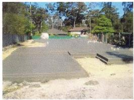
After all the rough in work is done and inspected, the concrete sub-contractor then is back on site to ensure compaction of the dirt, provide the required vapor barrier, termiticide, additional steel in the
