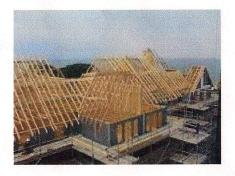
Your pre-manufactured roof trusses are then installed on top of the block wall/wall. The trusses are connected using specified connectors that are set into the concrete in the block. Roof sheathing is
